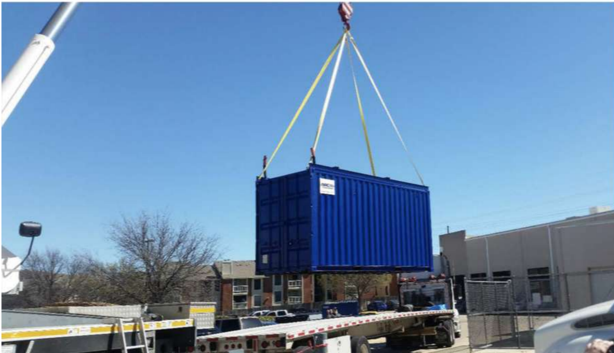
Image 6: Shipping the C3 Two using standard methods designed for ISO container movement.
