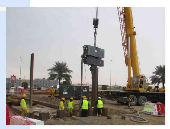
A vibro hammer is used to drive sheet piles or other elements into the soil by vertical vibrations. The adjacent soil particles are put into motion and thus soil is 'loosened'.
