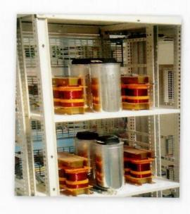
To ensure the preservation of maximum energy and power we designed and manufacture the automatic power factor correction panel which can improve the system power factor from poor to the target value in AC power distribution system by reducing the circuit loss while increase and improving the power output of the transformer.
