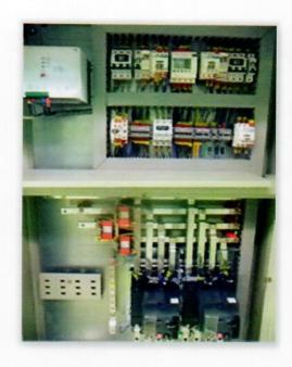
Automatic transfer switches are used to automatically transfer the main source to standby genarators on failure of the main source/supply. Upon the main supply is restored, the system automatically change back and stops the generator, after the short period of cooling down the standby generator set it will be eventually shut down.
